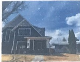
New homes, such as this single-detached home, are often larger when rebuilt (up to a maximum height of 3 storeys or 11 metres and 45 per cent lot coverage).
